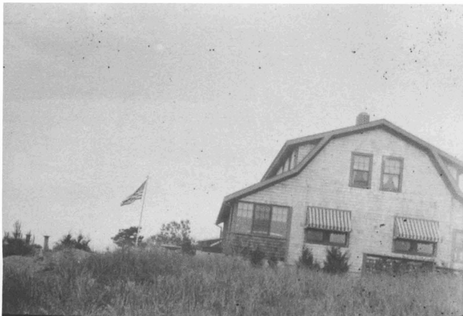
Fig. 2 Snapshot view of farmhouse from cove showing second dormer and gambrel roof, post 1931
